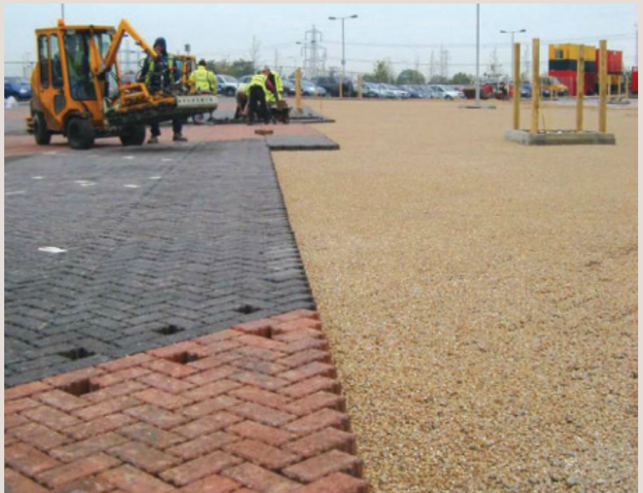
Figure 42: Machine laying of concrete paving units offers a particularly efficient solution for permeable as well as conventional block paving.
