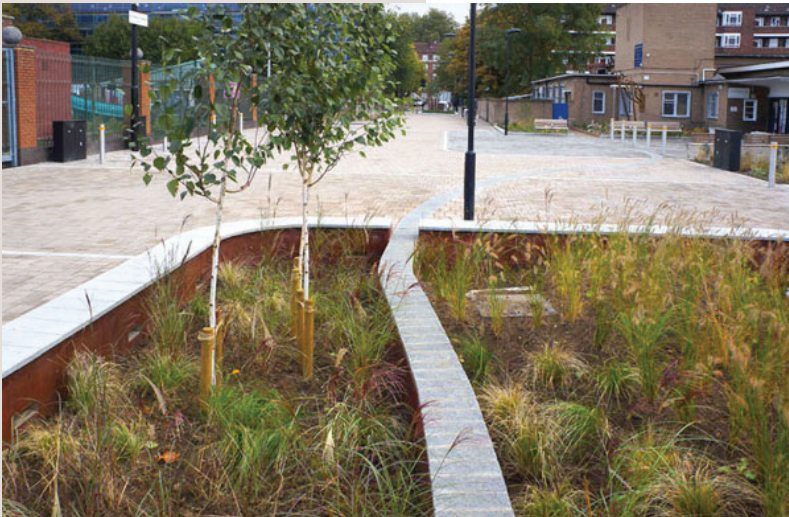
Figure 9: CBPP retrofitted over an existing road structure collects water and discharges it through slot drains into adjacent rain-gardens.
