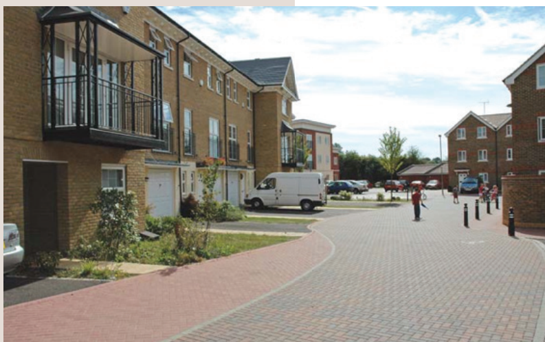
Figure 3: CBPP in a high density development.
